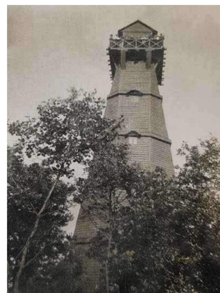
Abruca leading light rear lighthouse before renovation, picture from the year 1915
