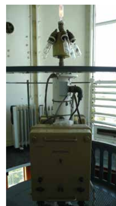
The lamp switcher with 1000 W halogen bulbs in front of a Fresnel lens, photo from the year 2009, photo V. Laitus
